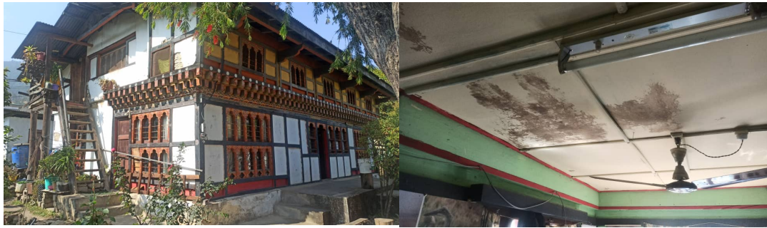
Existing condition of the Range Office
