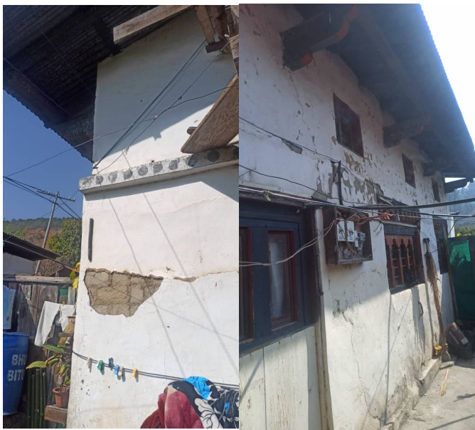
Existing condition of wall in Lobesa Range Office
