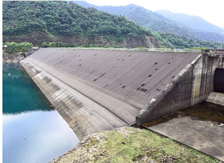
Figure 2 Example of a CFRF dam. Source http://www.allcons.de
