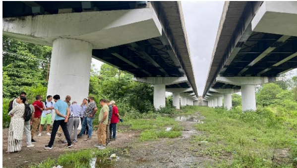
Elevated Road along Haridwar-Dehradun Highway within RTR
