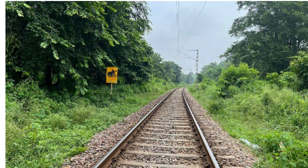
Railway track near Haridwar within RTR with precautionary signboard
