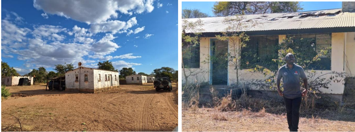
Plate 3: DNPW Staff houses at Lochinvar National Park
