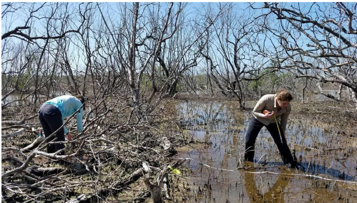
Figure 19 Mangrove damage from intense wind generated by Hurricane Irma three years after Hurricane Irma. Very little mangrove recovery is evident 104
