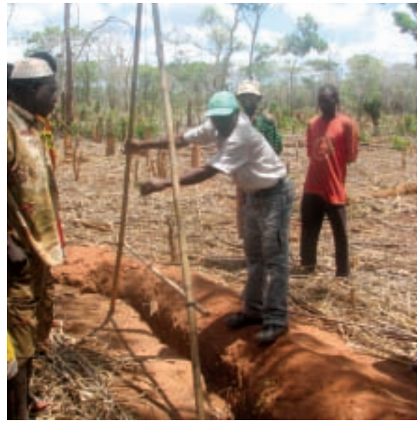
Laying out contour ditches in Quirimbas National Park, Mozambique. The ditches capture runoff during storms, increasing soil moisture and reducing soil erosion, so crop yields increase.
