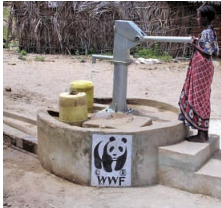
In the Kiunga Marine National Reserve in Kenya, hand pumps have been installed and wells have been covered in some villages to improve water quality.
