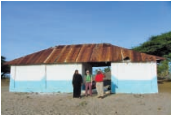
Health dispensary constructed by the community before the PHE project in the hope of attracting a nurse to Mkokoni village in Kiunga Marine National Reserve, Kenya. The building was used for mobile clinics at the start of the project.
