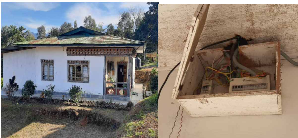
Figure 3: Existing Range Office, Damphu
