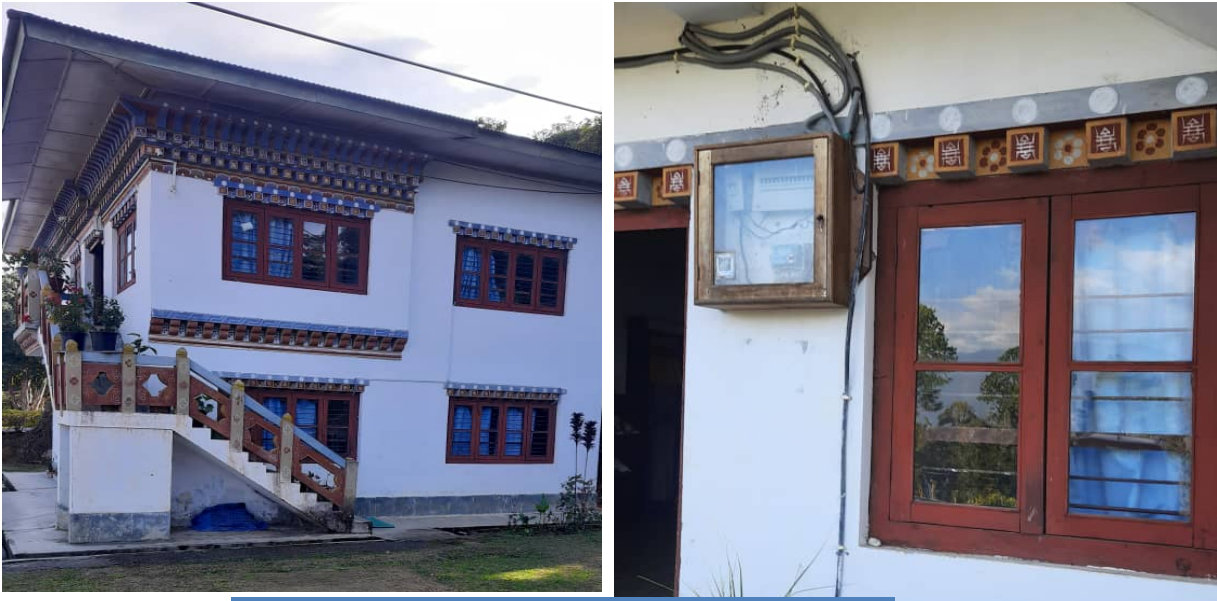
Figure 2: Existing Division Office, Damphu
