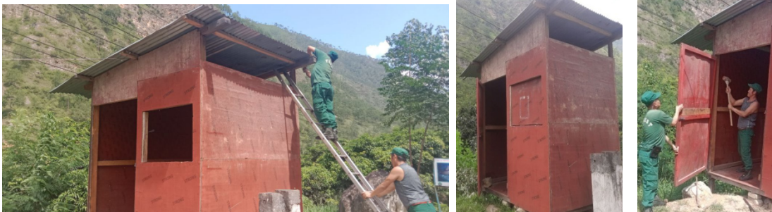
Figure 6: Dismantling of the check post made of plywood.
