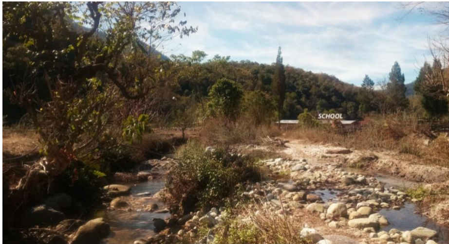
Figure 2 Location of school w.r.t. the eroded river bank
