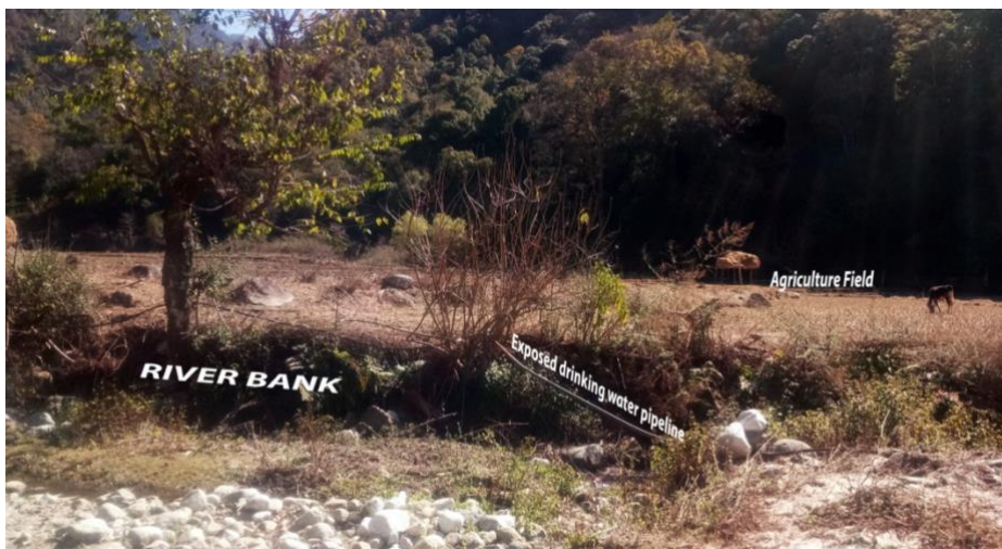
Figure 3 River bank protection site
