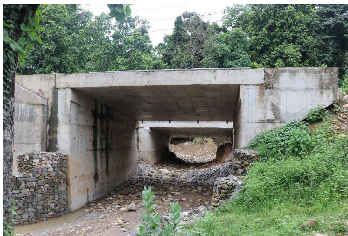
An underpass being constructed at N-B road (©Swarnima Shrestha /WWF Nepal)
