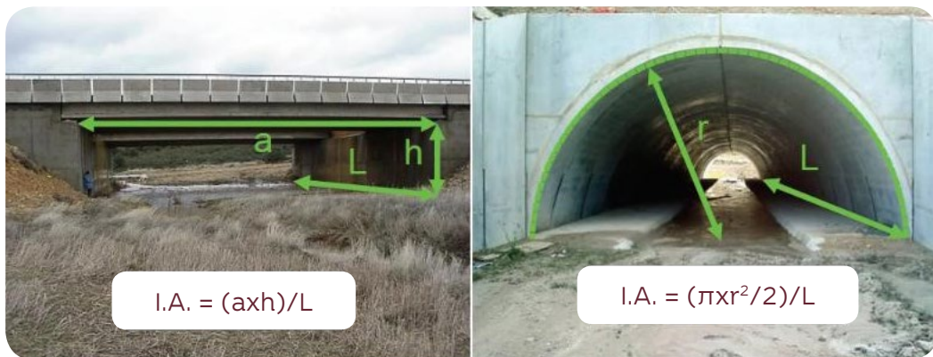
Figure 10. Opening index in a quadrangular structure and in a circular section structure
