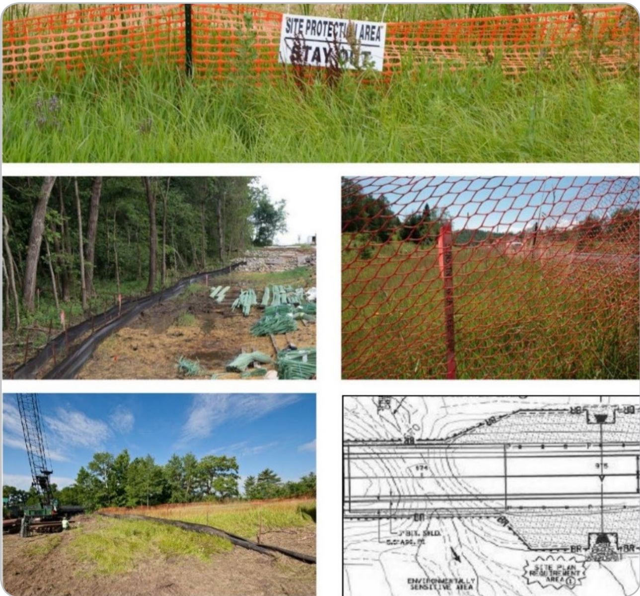
Figure 7. Examples of mesh fencing used as adaptations for wildlife crossings.
