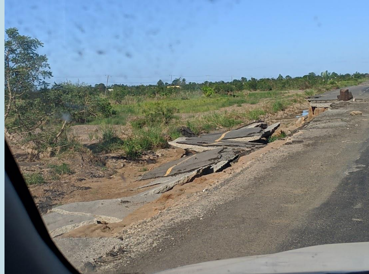
Image credit: D. Nelson, use of substandard materials - Mozambique
